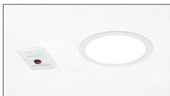
Standard test switch shown installed
