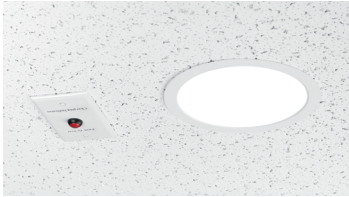
Standard test switch shown installed
